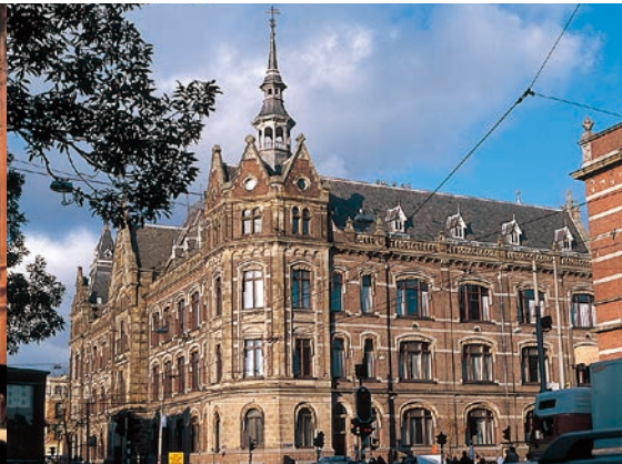
Konservatorium Amsterdam (Netherlands)
