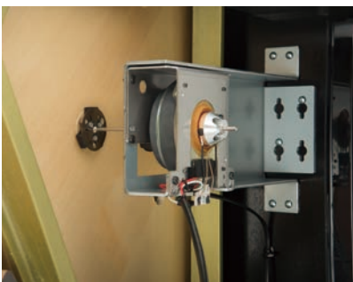
TA2 type control panel
